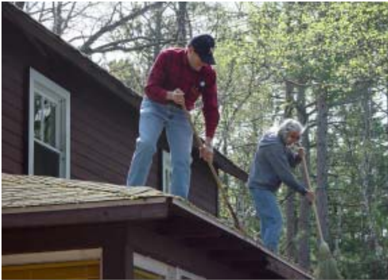
Jim and Mary Kelsey sweep the roof of the Lodge.
